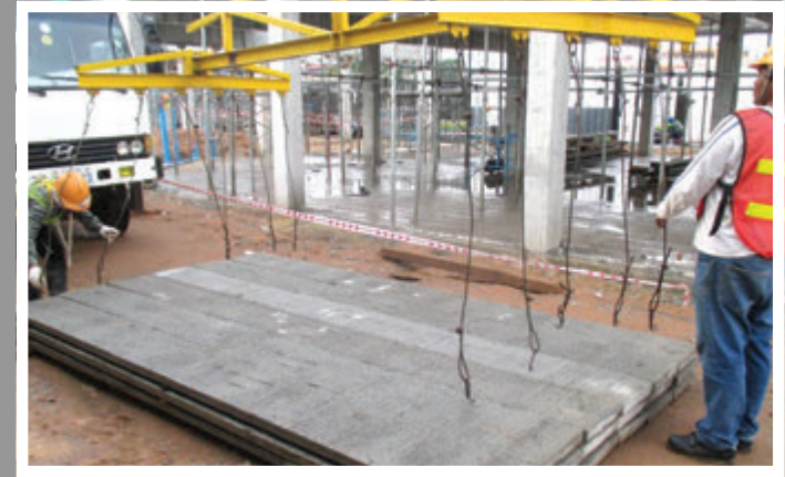
CPAC Plank Slab Installation
