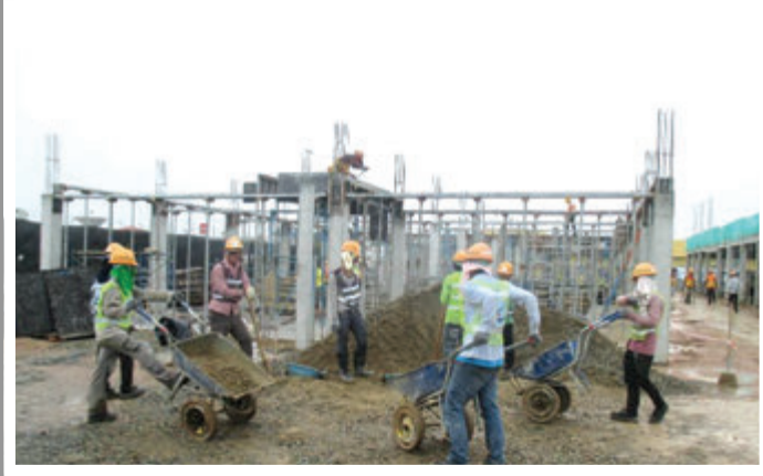
Crush Stone Compaction for Slab Concrete Casting
